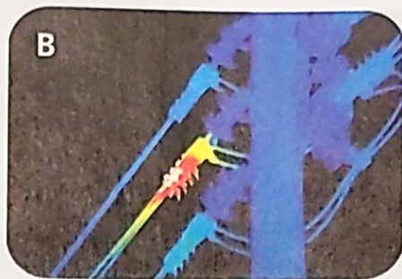
Figure 12 A thermogram can be used to diagnose problems in a utility line. A When viewed in visible light the wires all look the same. B The colors in the thermogram image show that the electric current in the center wire is not flowing as it should.
